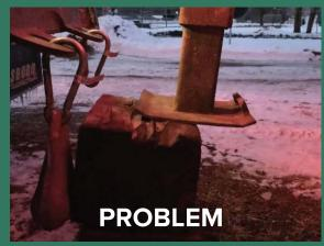
Wind caused jack to slip off wood block
